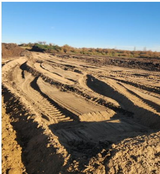
Above: It took 88 dump truck loads or 1,110 cubic yards of granular material to fill the peat hole.
