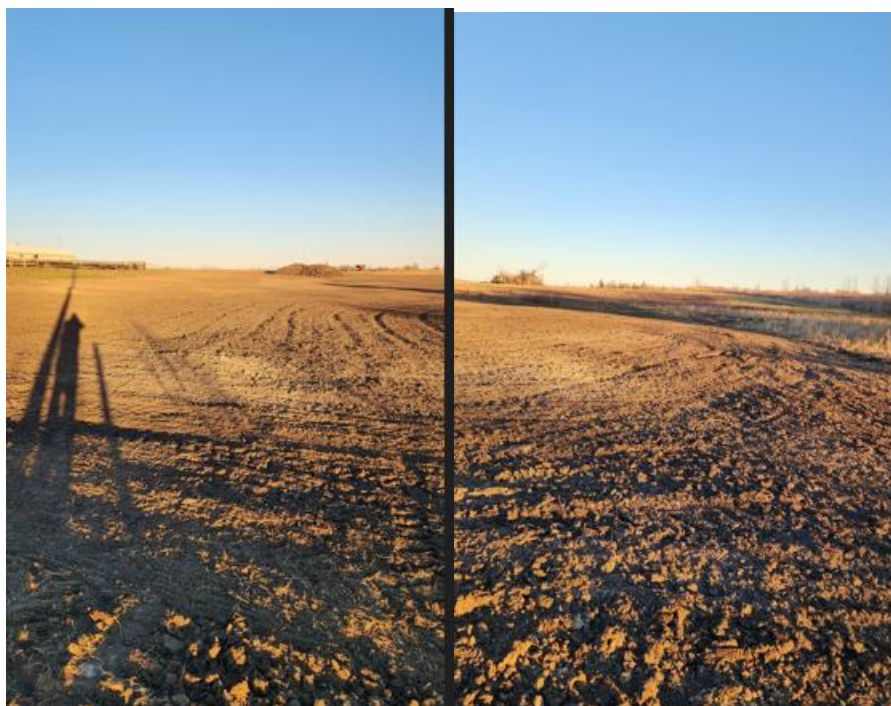
Above: It took 88 dump truck loads or 1,110 cubic yards of granular material to fill the peat hole.
